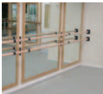
Wall-mounted brackets and end brackets installed at Essex Dance Theatre, Chelmsford.
