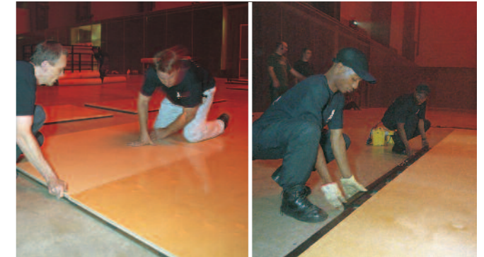
Installing the panels
