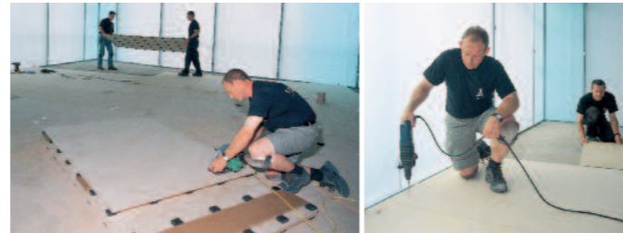
Fitting at perimeter
