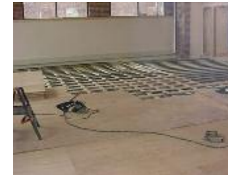
Installation of Harlequin WoodSpring at the Boston Ballet School
