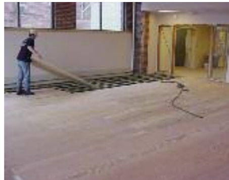
Completion of first and second layers of basketweave structure
