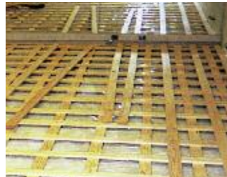
Installation of third layer in progress
