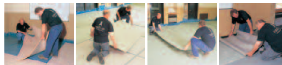
Cellular polyurethane layer First layer of semi-flexible panels Top semi-flexible panel layer with joints staggered Harlequin vinyl performance surface
