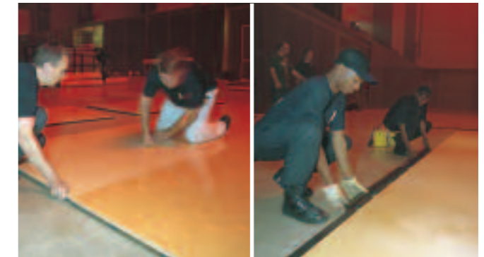
Installing the panels
