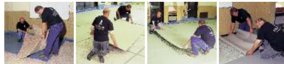
Cellular polyurethane layer First layer of semi-flexible panels Top semi-flexible panel layer with joints staggered Harlequin vinyl performance surface
