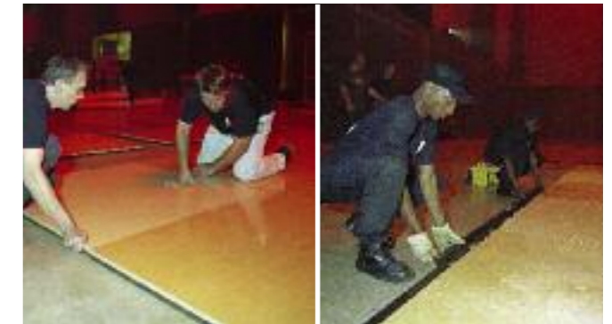
Installing the panels
