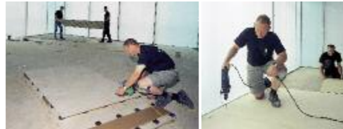
Fitting at perimeter
